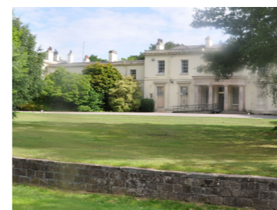
The ha-ha which is invisible from the house.
